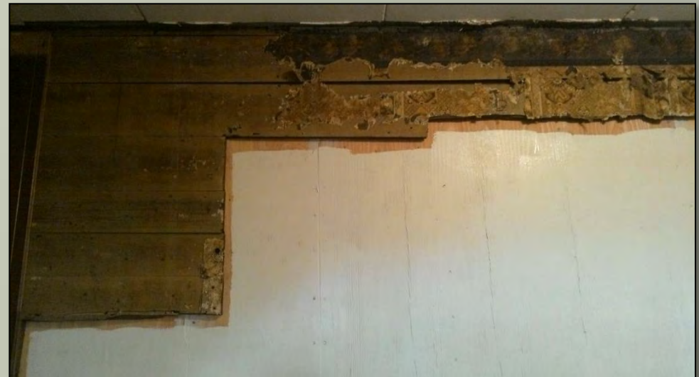
South wall closed and remaining siding and historic wallpaper reinstalled
