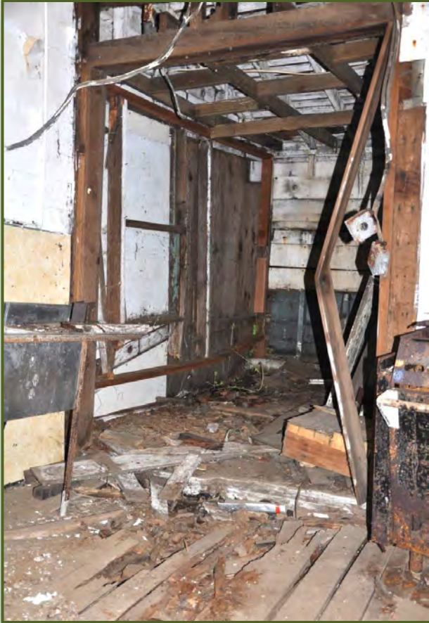
Rotted kitchen floor from past flooding, collapsing shed additions, and buckling walls
