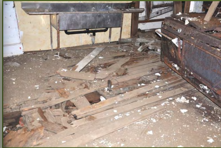
Rotted kitchen floor from past flooding, collapsing shed additions, and buckling walls
