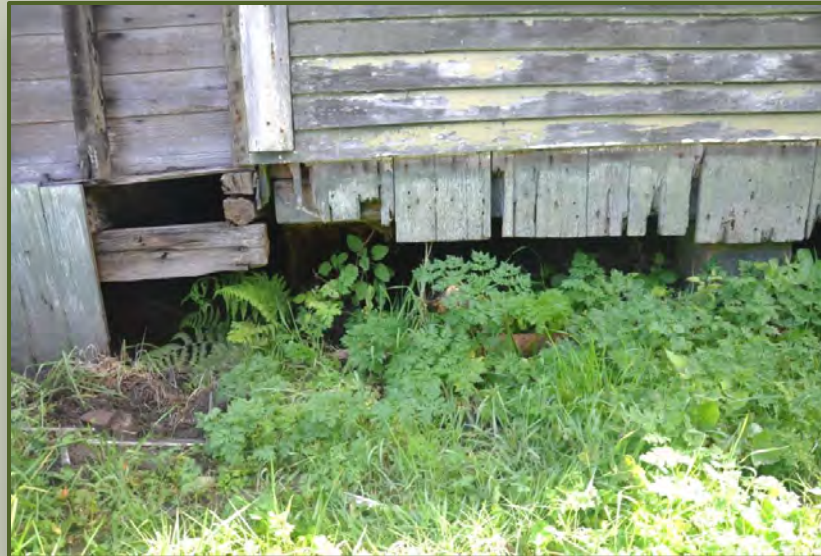
Foundation structure completely rotted away
