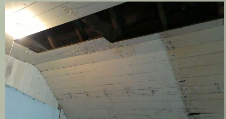
Ceiling closed and lead paint abatement continues upstairs through individual rooms and hallway
