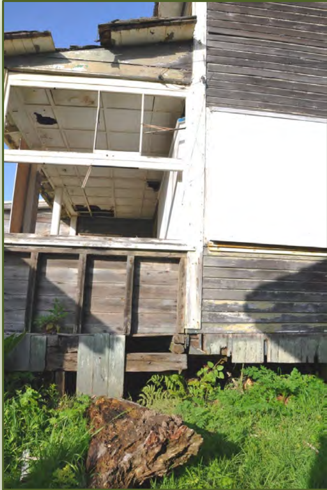
Foundation structure completely rotted away
