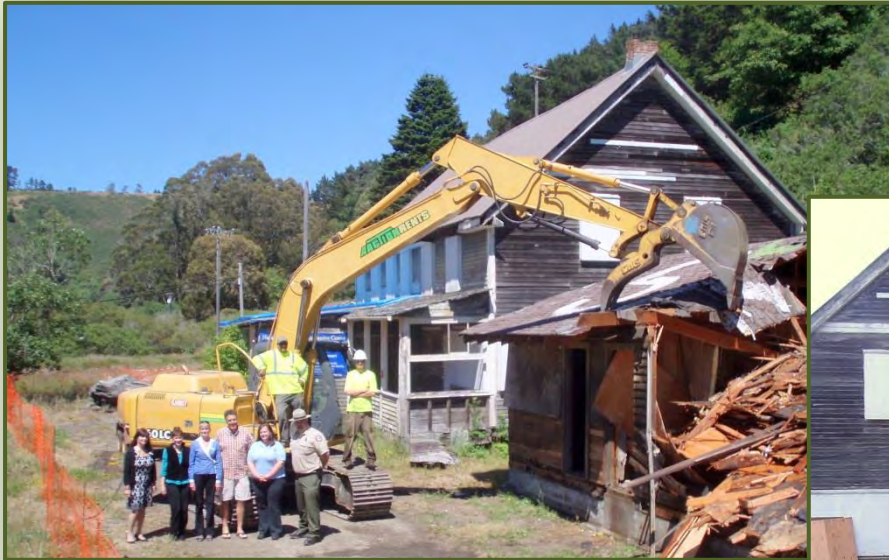
Demolishing motel building and dismantling brick chimney
