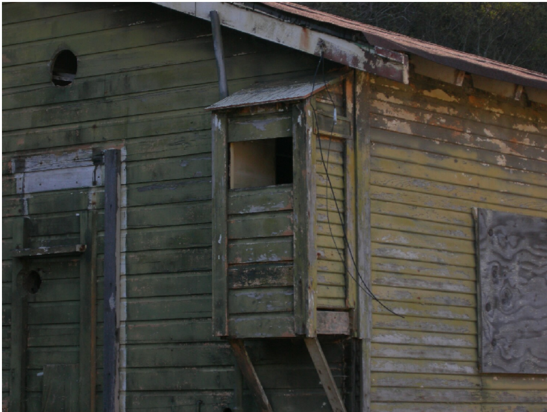
Fig. 2. East Cottage California Cooler after reconstructi on and modification to strengthen, make more watertight, and improve access for C. townsendii.
