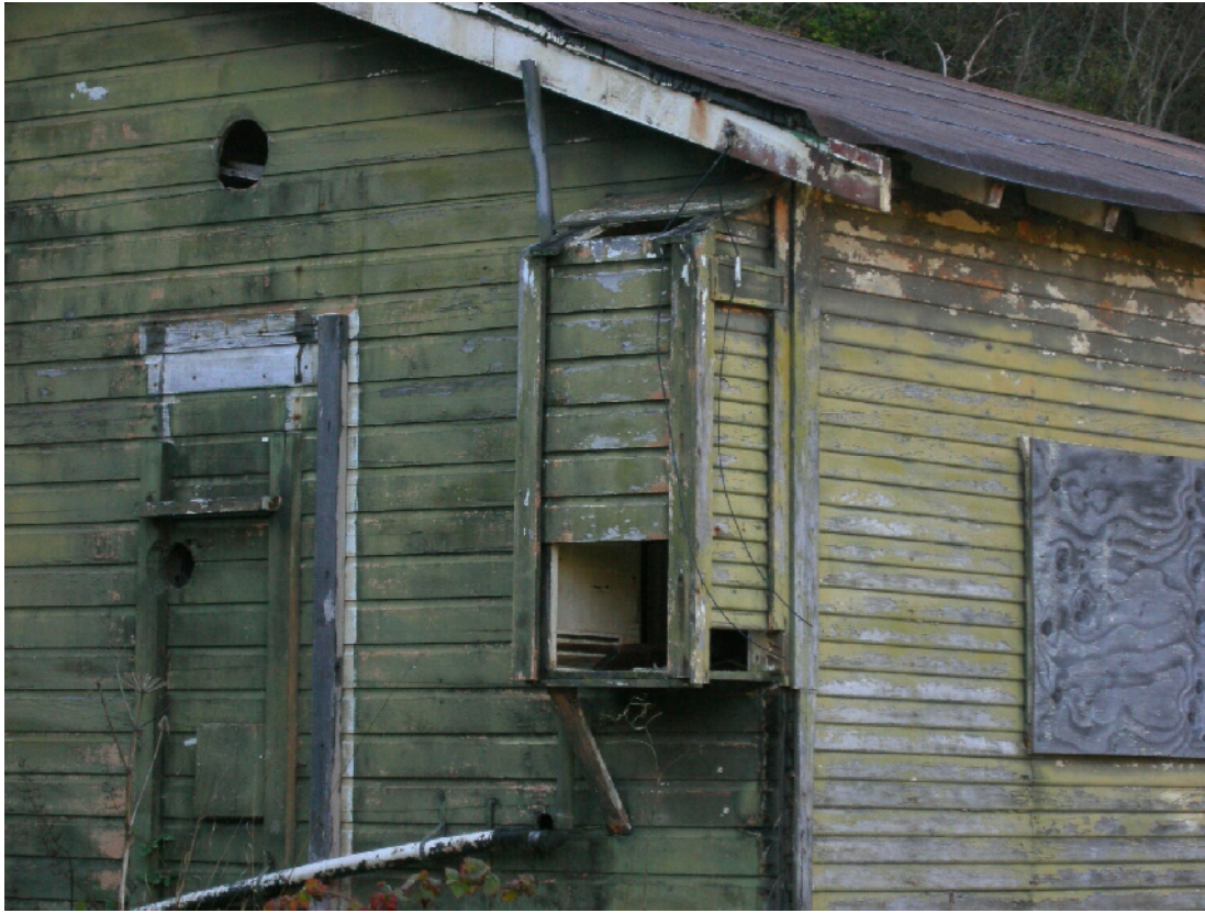
Fig. 1. Example of prior condition of California Cooler, East Cottage. Roof missing, structure failing, openings at bottom provide easier access and viewing by public.
